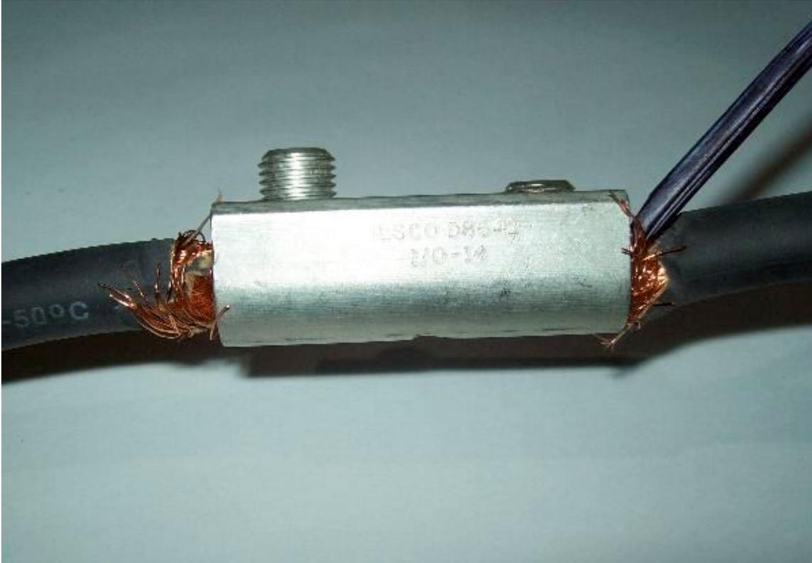
**This is the aluminum connector/reducer to attach wires with. Just be sure to spread liberal amounts of Di-Electric grease on the bare wires before inserting them into the connector and be sure to screw them down real tight for a proper connection.**
