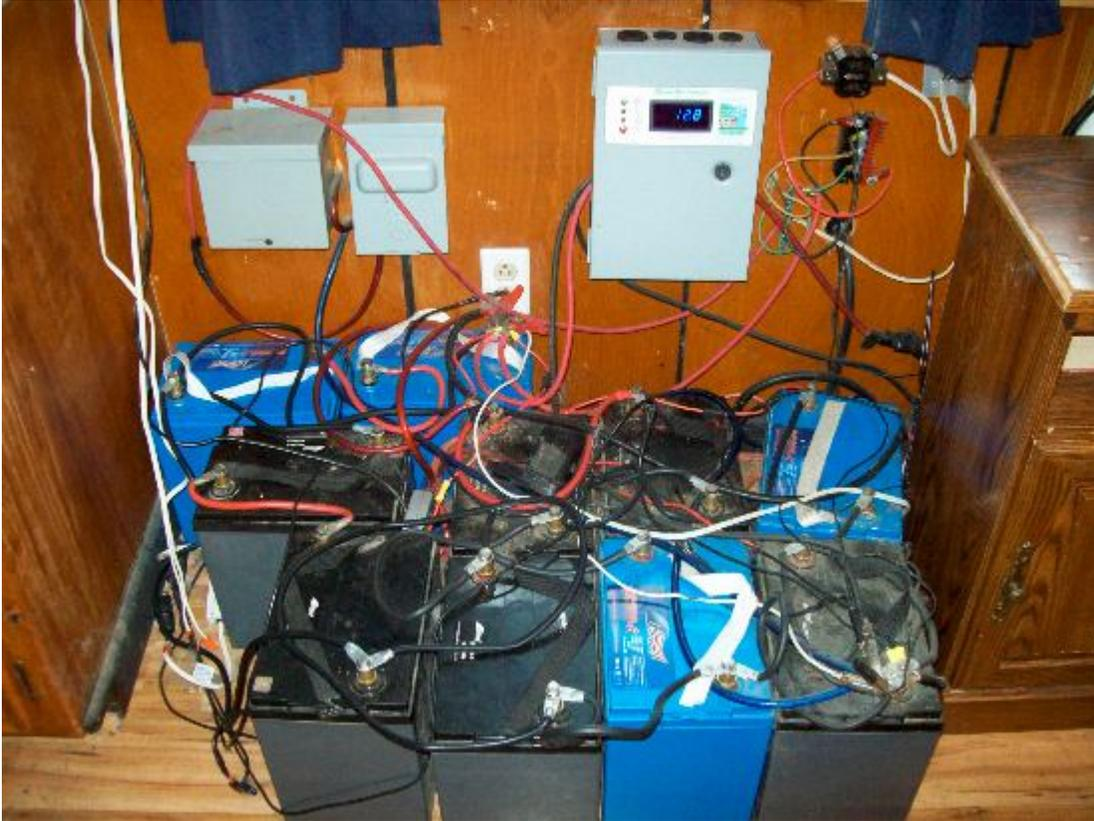
**Here are my 10 AGM 250 amp 6 volt batteries, that give me a total of 1,250 amps to draw from. Yes I agree this looks ugly but note (the table lamp in the above photo is sitting on a desk). That desk pushes up over these batteries and they are well hid and only the charge controller peeks above the back of the desk when you get close to it. This way my wife is happy, I'm happy, were all happy. And we love our 12 volt power.**
