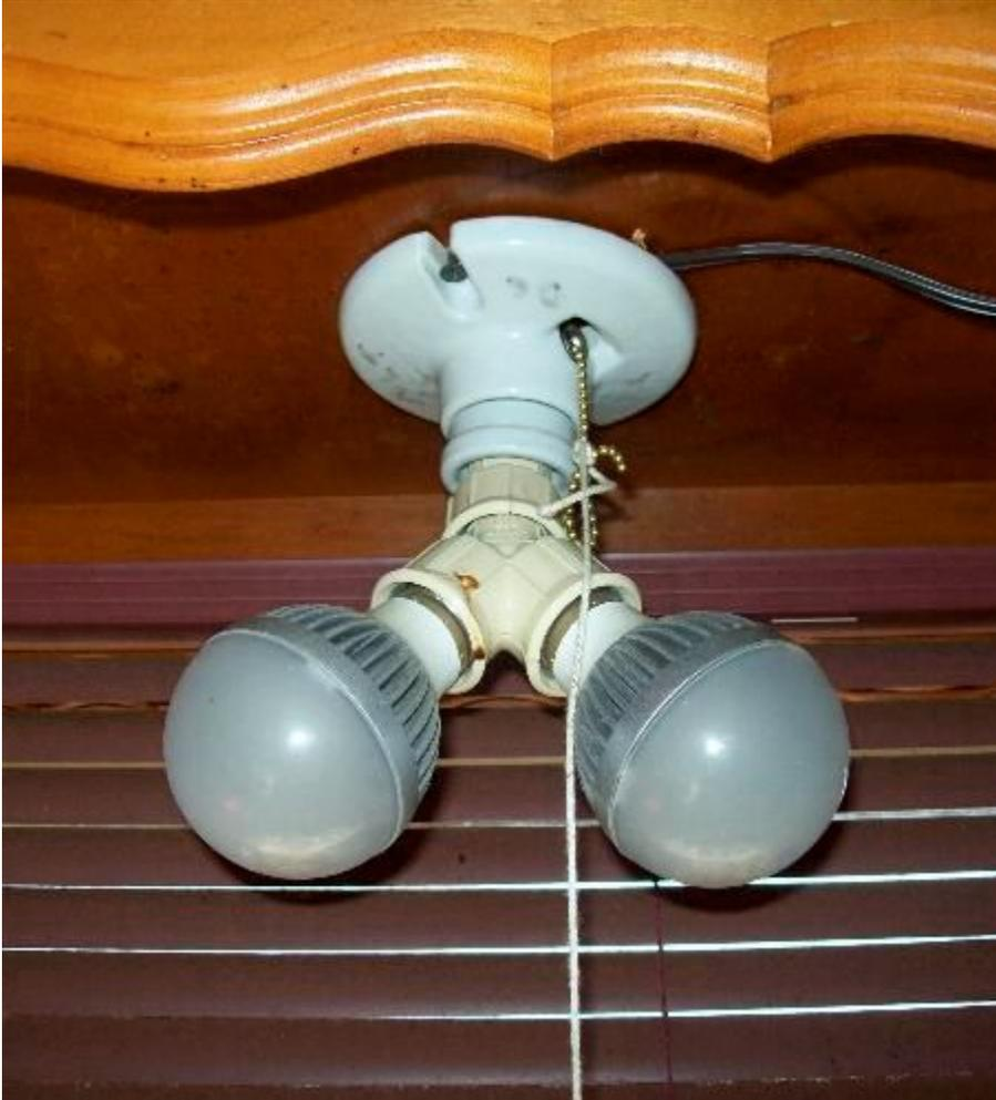
**This is a 110 volt AC fixture with a Y adaptor and I have 2 – 12 volt lights bulbs 45 watts equivalent light each but they only use 5 watts of power each – NOT 45 watts each. Note the pull chain for the on/off switch.**
