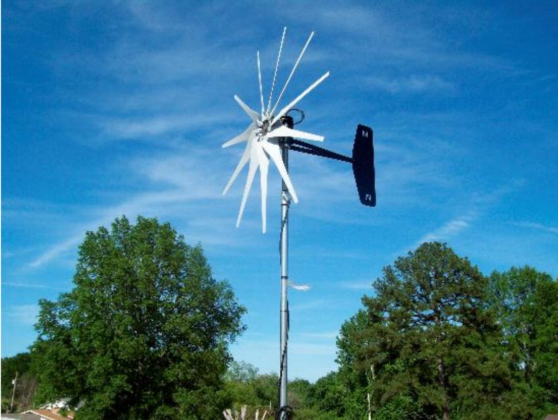
**My wind turbine; we don't get much wind here in Arkansas but I wanted an alternative charging method to my solar panels. And I am ever so happy I choose the Wind Blue Power Low speed PMA (Permanent Magnet Alternator) as it starts producing 12 volts in just 5 MPH wind. And it produces 13.5 volts in just about 6 ½ MPH wind.**
