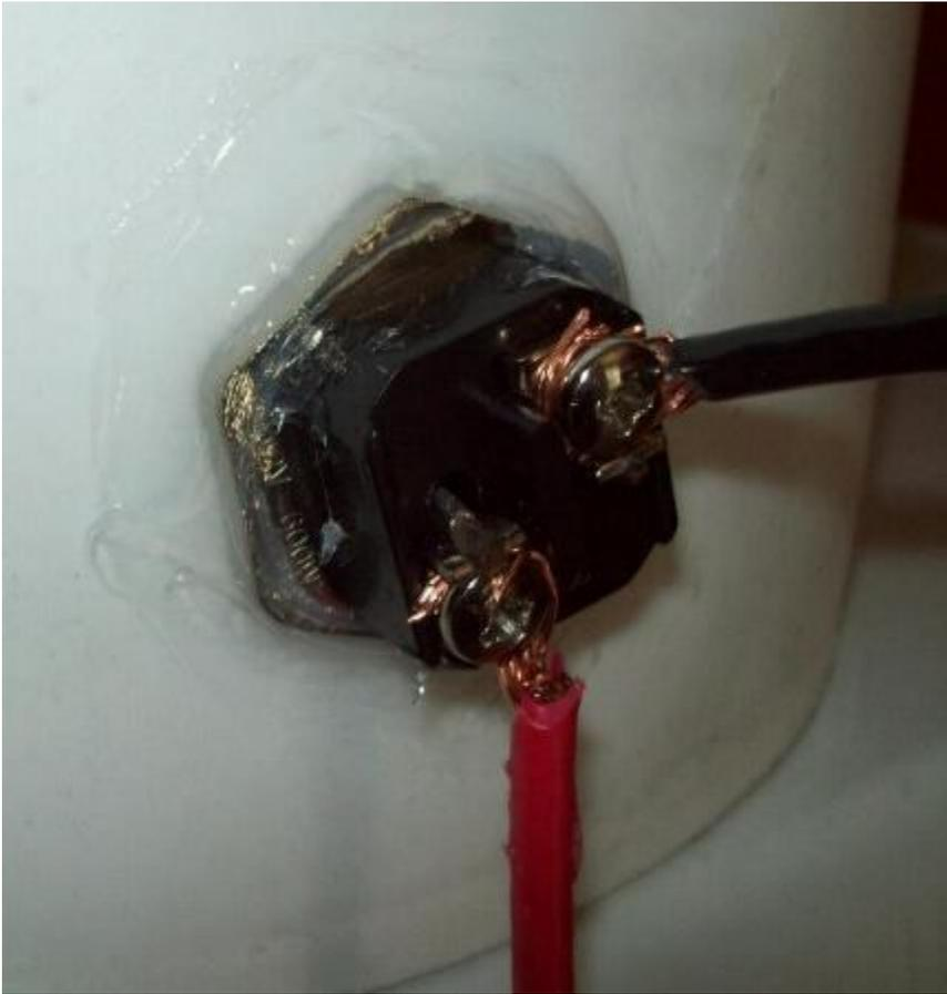
Be careful when attaching wires to the heating element as you do not want to break the seal formed by the Aquarium sealer. Also note how we goop on the aquarium sealer. The reason you use Aquarium sealer is regular silicone has chemicals in it that can leach into your water, so don't be cheap, USE Aquarium sealer. After the Aquarium sealer dries thoroughly you disconnect your solar panels and disconnect your wind turbine, so you can hook up
